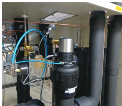
*The temperature control units are supplied fully encased. The fittings are generally placed at the top, with threaded or flanged connections according to size. In this way, the 4 sides are fully accessible for any maintenance, assuring the utmost freedom of installation and orientation in utility rooms, even in narrow spaces.*
